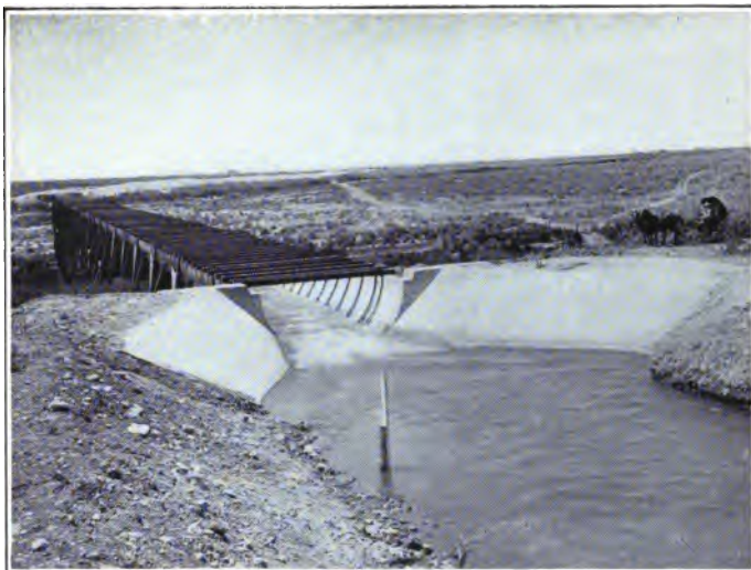
METAL FLUME FOR CONVEYING WATER ACROSS DEPRESSION ON BOISE PROJECT, IDAHO.
